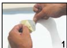
1 Remove the protective paper from the self adhesive flange
