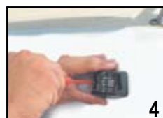
4 Screw until the rawl plugs are secured
